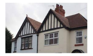
This pair of houses on Glenmore Road illustrate the impact of replacement widnows and roof covering (right) as compared with the originals (left). Concrete tiles have a harsh stepped appearance. The decorative finial and subtle pattern of lapped ridge tiles have been lost. The replacement uPVC windows are flat and lacking in the attractive modelling of sashes with horns, cill and cornice detail and vertical rhythm of sash boxes.
