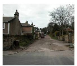
Arno Road West of Fairview Road is unmade, but heavy use has lead to the creation of potholes and some uncoordinated patch repairs
