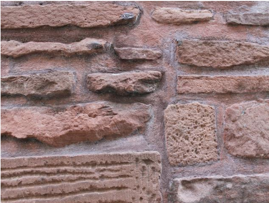
Photo 2: pointing slightly recessed with surface of stone.
