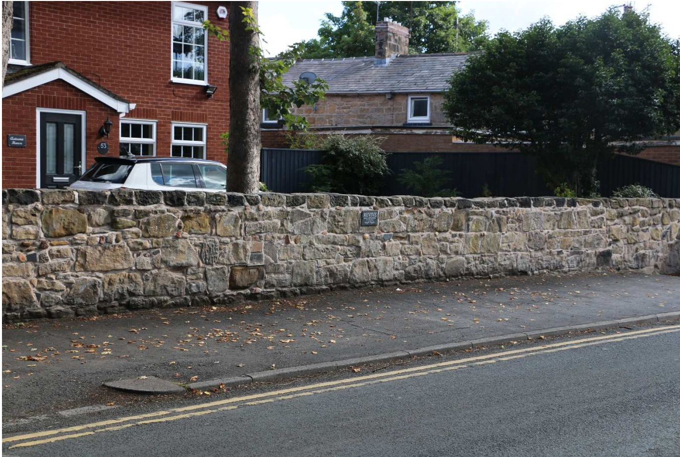
Fig. 26 Sandstone wall restoration on Rose Mount: example of good practice
