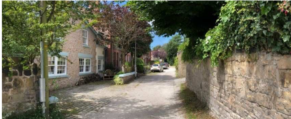
Fig 2. Sandstone walls on Hughes Lane
