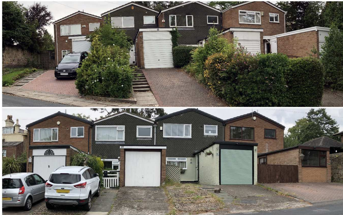
Fig.6 Houses on Fairclough Lane (below) and Rose Mount (above) referred to in 1978 report
