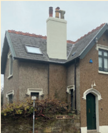
David and Elizabeth Coombes , 1 Mount Pleasant for the complete re-building of a very prominent chimney stack, including reinstatement of original pots.
